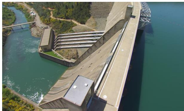
The Shasta Dam in California has been generating power since 1945
