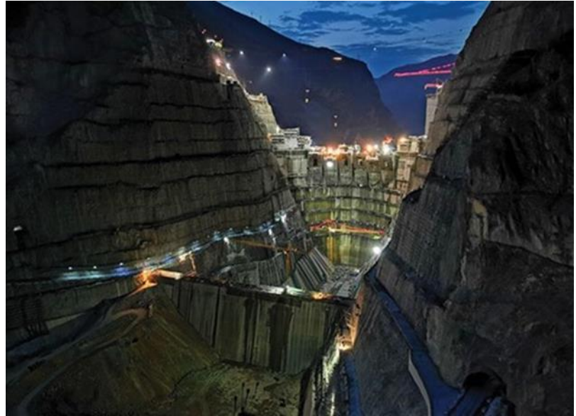
Wudongde project construction at night
