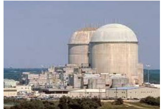
Comanche Peak Nuclear Power Plant Photo Credit: NS Energy
