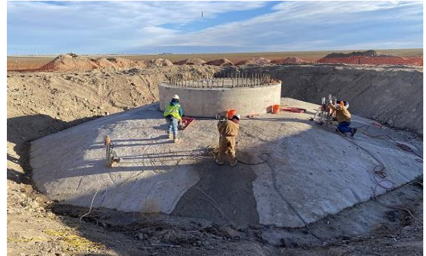
Foundation / Pedestal / Core Drilling – Niyol Wind Farm Photo Credit: Jack Harold
