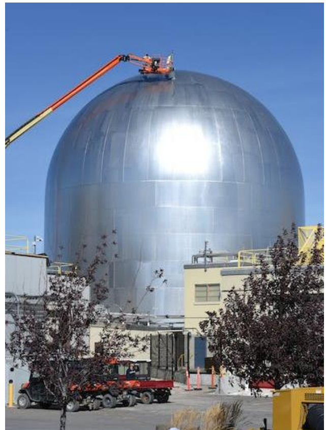
The Experimental Breeder Reactor-II dome receiving internal and external improvements in 2020.
