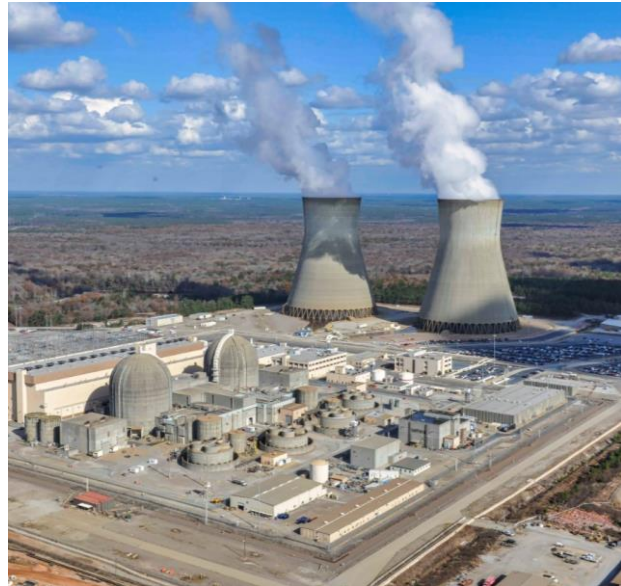
Westinghouse's AP1000 Reactors are currently operating near Waynesboro, Georgia at Plant Vogtle. The design is a two-loop pressurized water reactor that is touted as using a simplified, innovative, and effective approach to safety. Image Credit: SouthernNuclear.com
