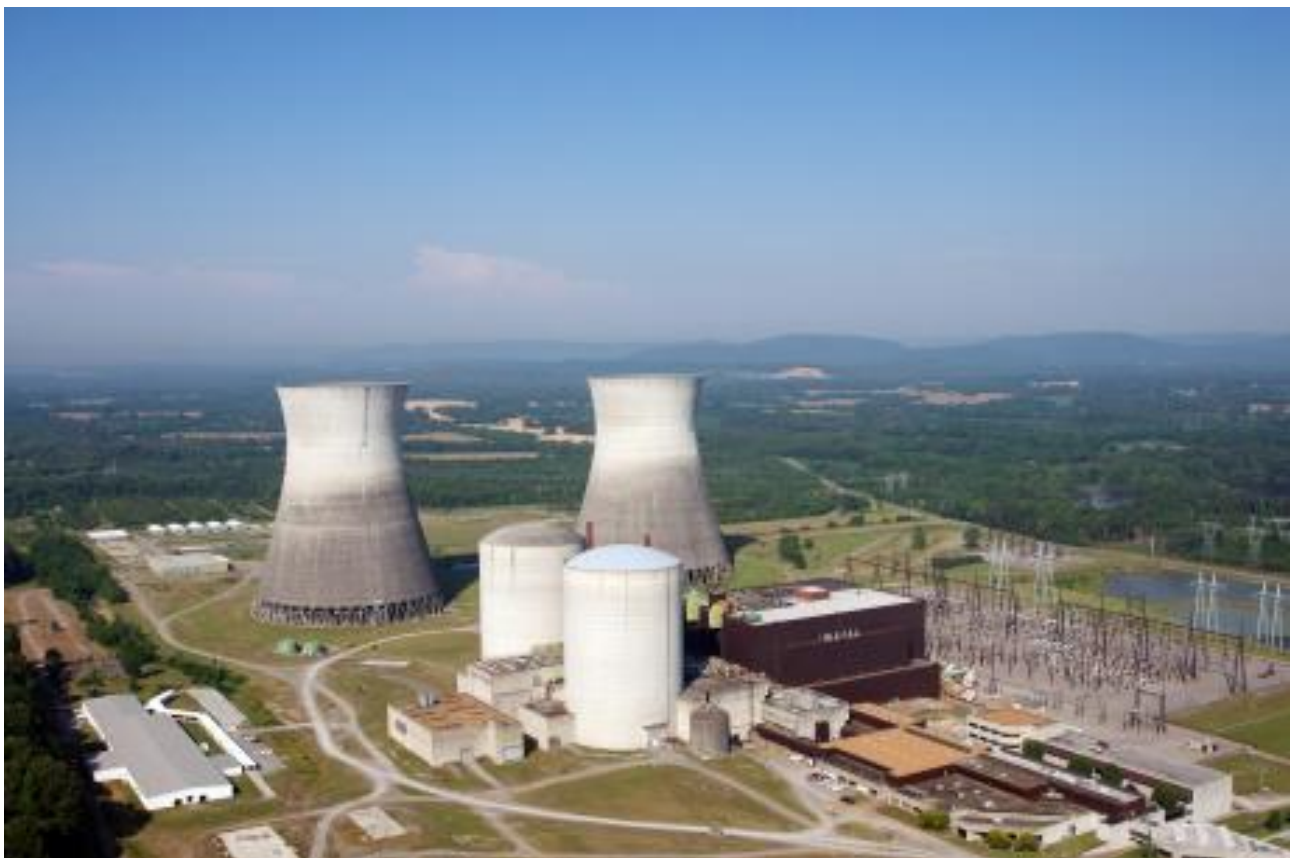
Bellefonte Nuclear Power Plant Site Image Credit: TVA
