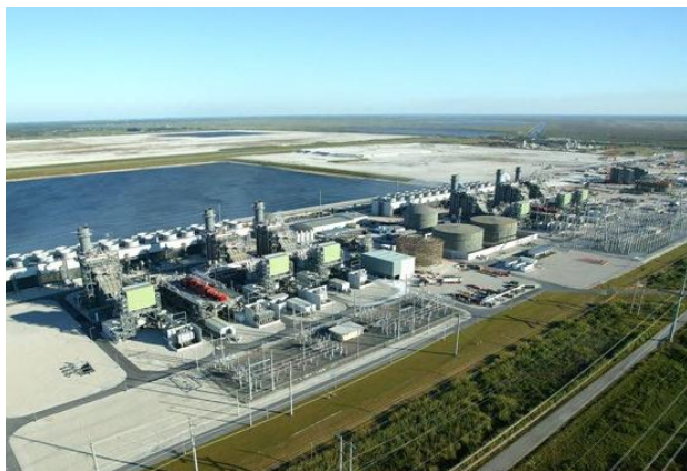
West County Energy Center in Palm Beach County is the largest U.S. natural gas power at 3,750 MW Image Credit: FPL.com
